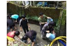
Sediment removal works at weir
